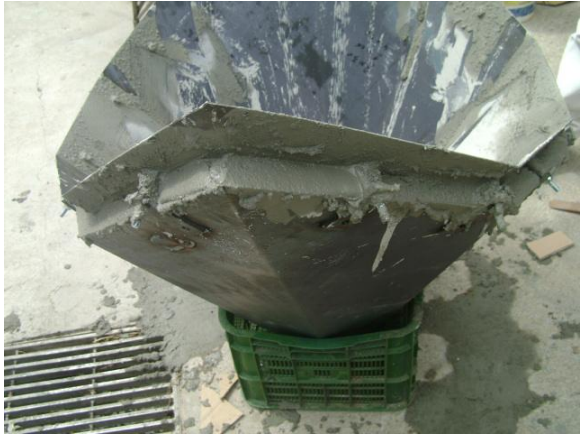
Fig. 8 – Mold filled with concrete mass
