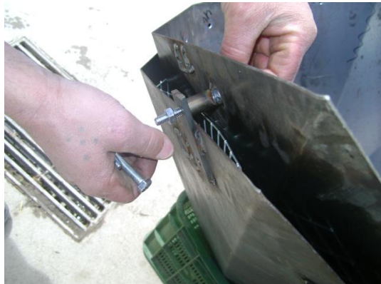
Fig. 7 – Jointing the funnel pieces
