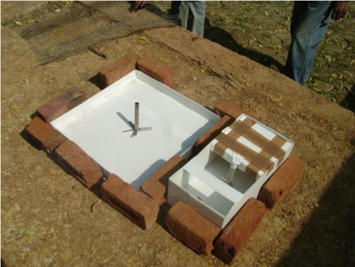
Fig 13- Molds for the basement and middle pieces
